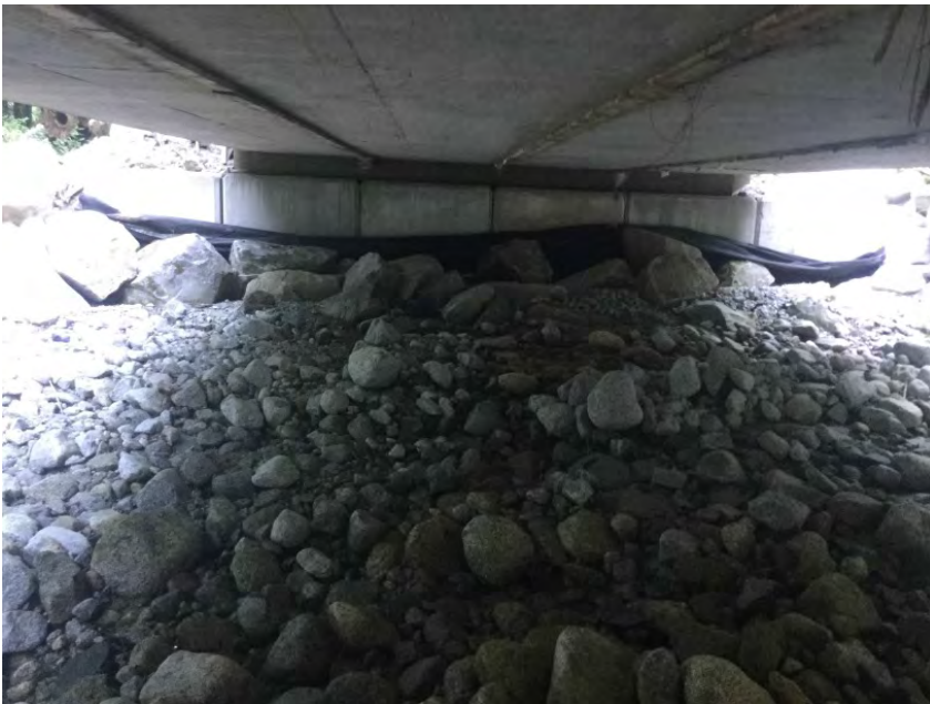
Right Bank Abutment
