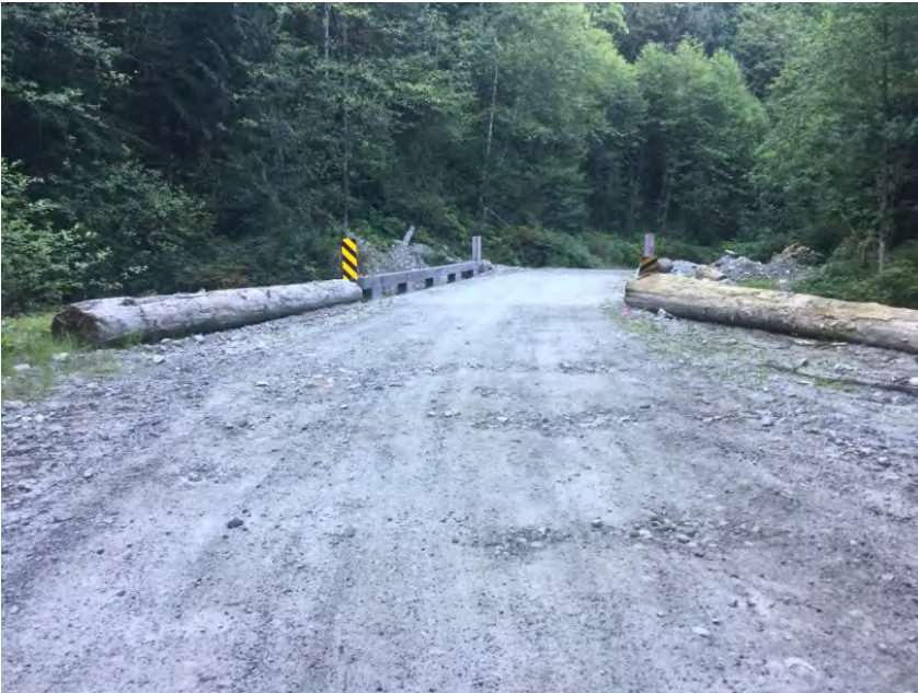
Right Approach Facing Bridge
