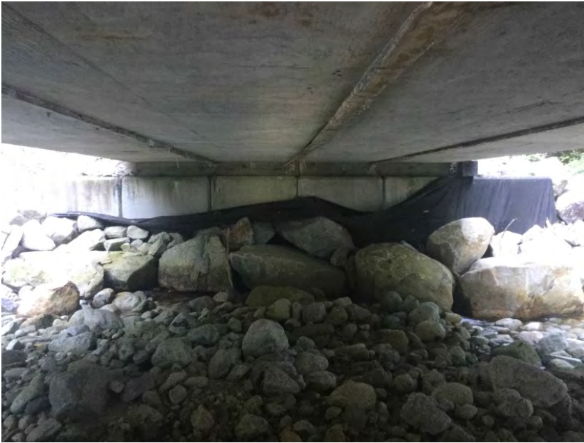
Left Bank Abutment
