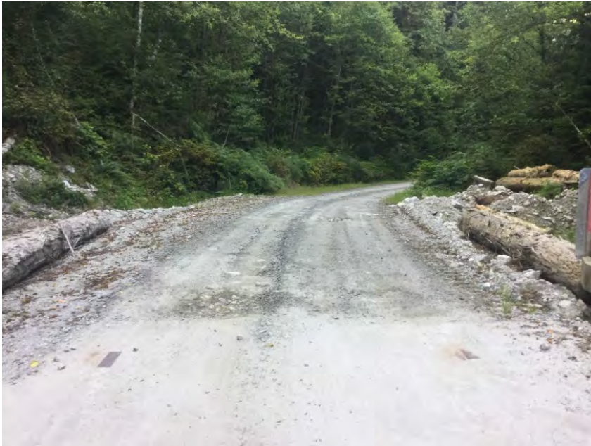
Left Approach Facing Away From Bridge
