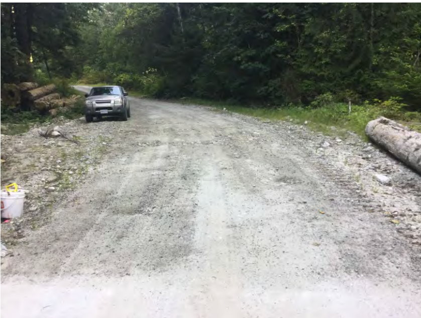
Right Approach Facing Away From Bridge
