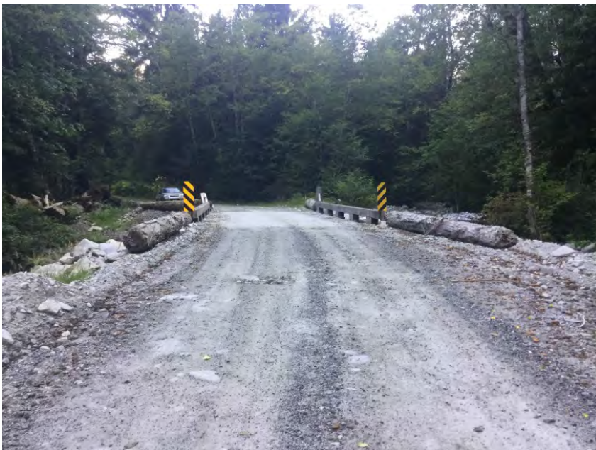
Left Approach Facing Bridge
